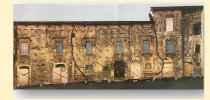
As required from the operators, the dispersions must be applied on the mortar in *a single treatment,* so we decided to apply the *aqueous nanolime suspension* by *aerograph nebulization*, by considering different Ca(OH)<sub>2</sub> concentrations.
